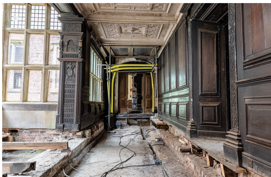
The east wing of the Gallery Corridor after the floorboards were removed Photo: Dave Brogan
